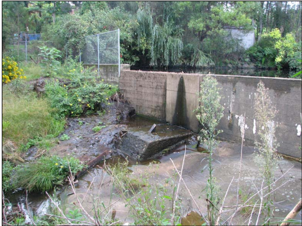
Plate 9: Dam 2 wall facing north.
