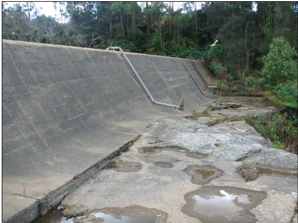
Plate 8: Dam 1 wall facing north.
